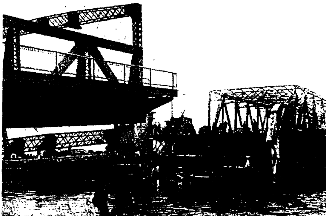
Figure 5-9 The wrecked east leaf of the Hackensack River bascule on the Lincoln Highway in New Jersey. In the left foreground the undamaged west leaf is shown in the closed position. At left (the north side of the wrecked leaf), the tailpiece and operating rack protrude from the waters of the Hackensack River. ( ENR. )
