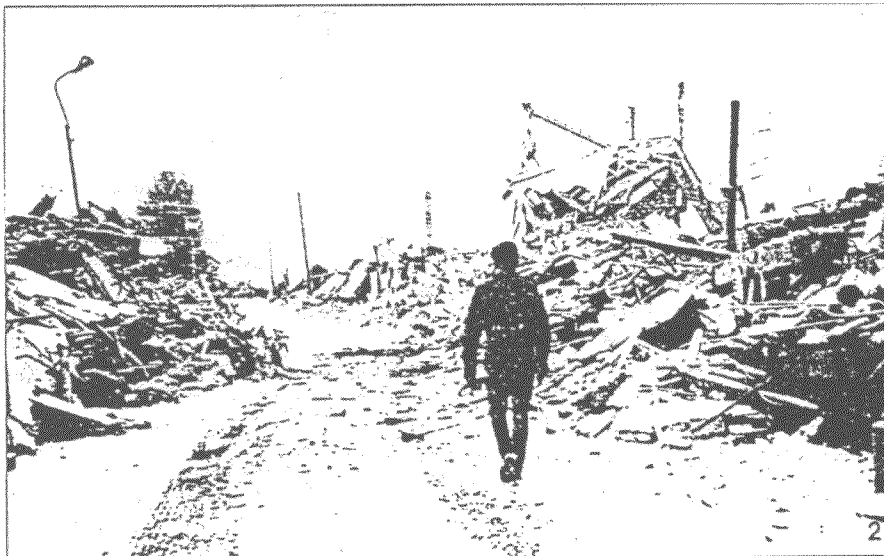
FIGURE 2. Main street in Nalband showing complete collapse of all buildings. Note complete collapse of precast-concrete frame school building on right side of street.
