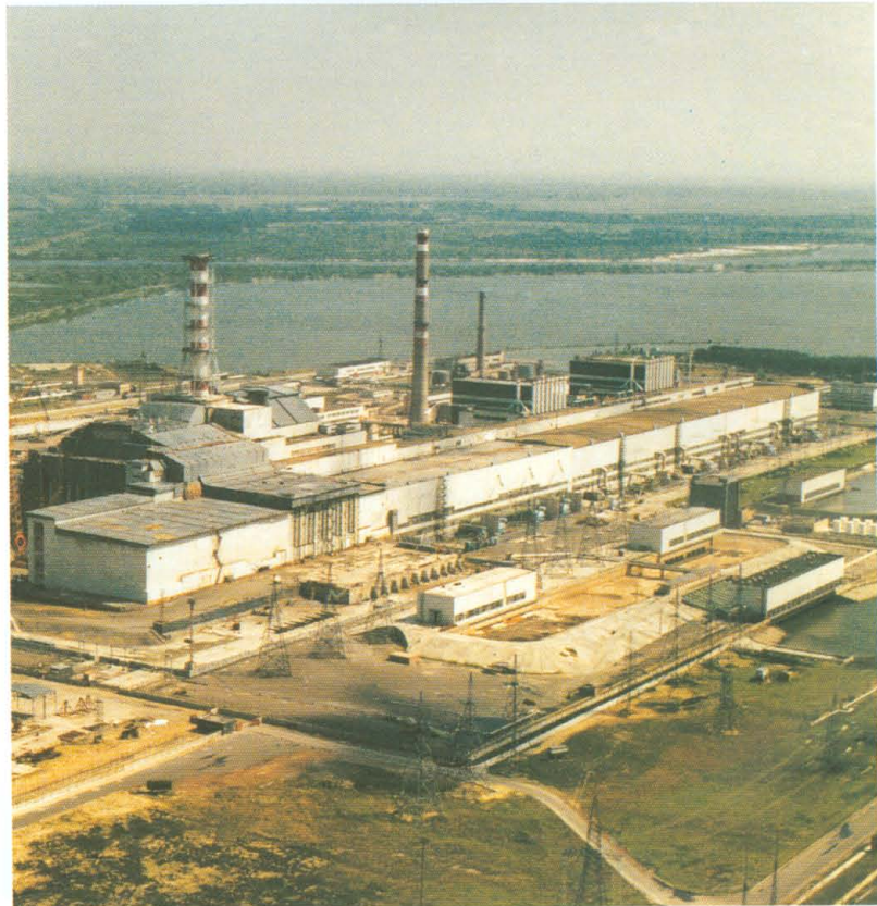
Units 1,2,3 and 4 of Chernobyl nuclear power plant. The Sarcophagus over Unit 4 is in the foreground credit:Mouchkin/IAEA
