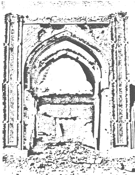
Behaviour of old building in earthquake of 1968 in Ferdous (Iran) September 1968
