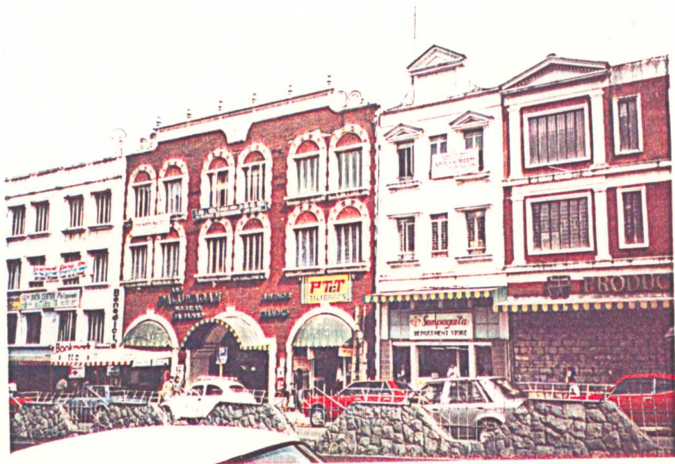
Photo 4.33 Historic townscape of Centre of Baguio City along the Session Road, lightly damaged.
