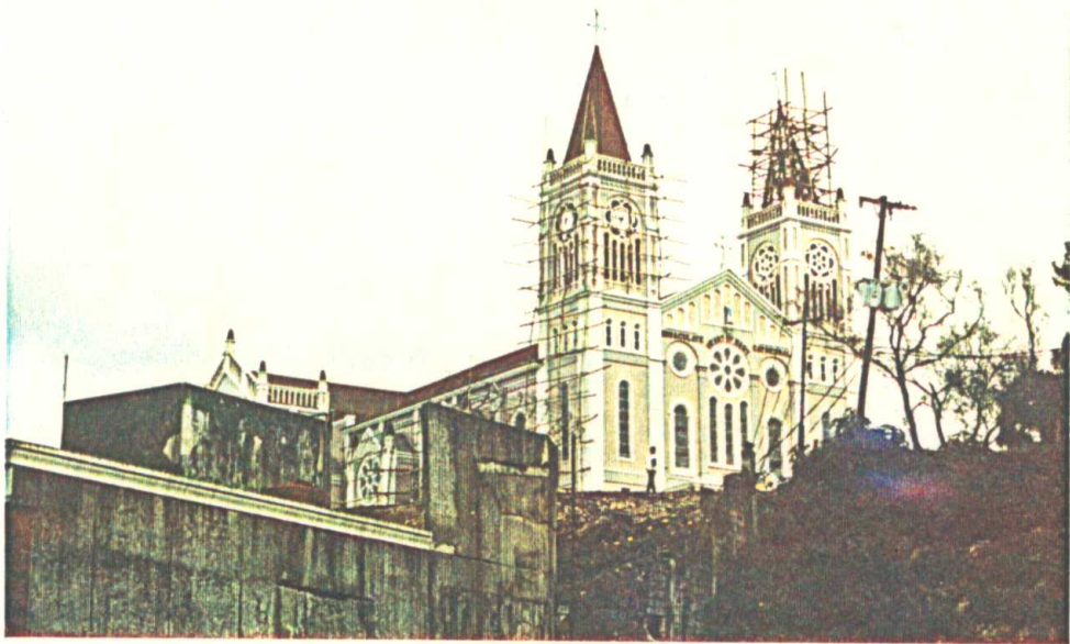
Photo 4.34 Cathedral at baguio City, damaged towers and failure of right side tower indicates dominant frequency content of the earthquake ground motions in Baguio.
