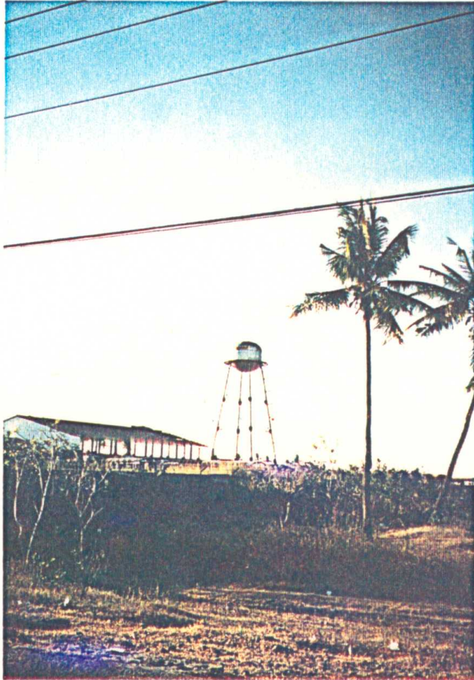
Photo 4.24 Elevated steel water tank near Dagupan City. No damage reported, could be attributed to specific frequency content of earthquake ground motions.
