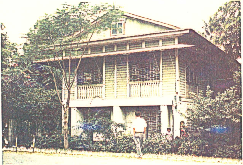
Photo 4.4 Typical larger timber-framed house of early 20th century. Such buildings suffered very very little damage (same damage from the flexing of the structured frame).
