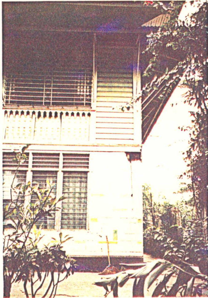
Photo 4.5 Minor cracking to masonry walls enclosing timber framed house - timber frames flexing in the earthquake caused damage to the stiffer masonry. Damage and failure could be expected at larger earthquake intensities.
