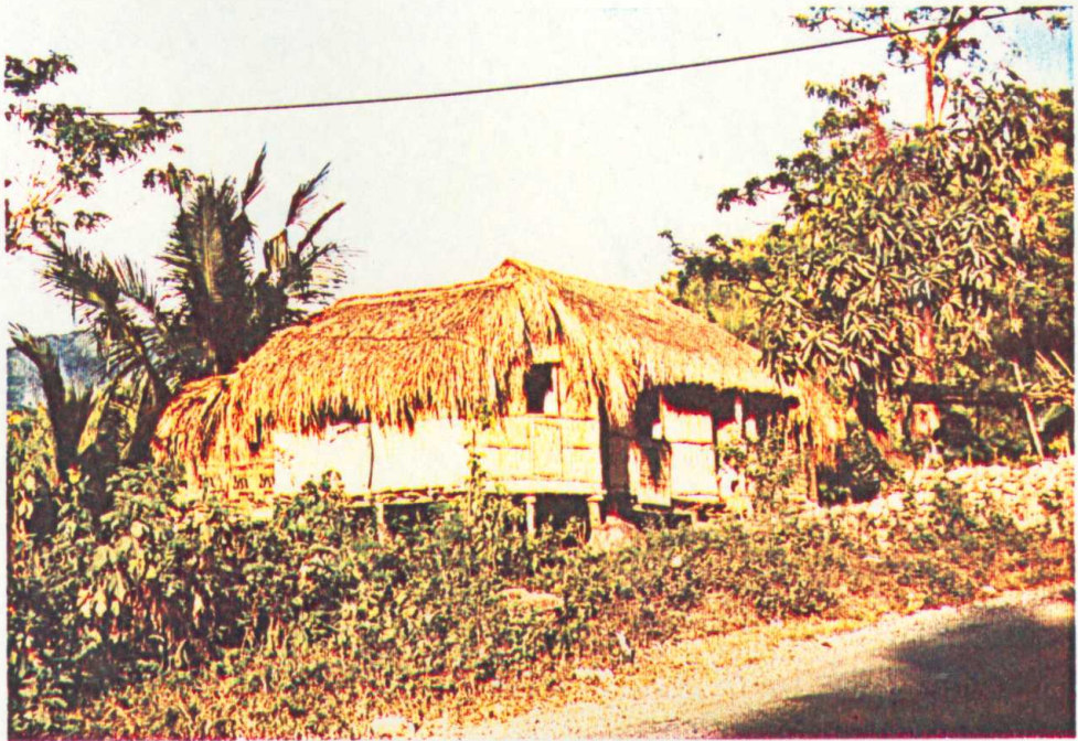
Photo 4.1 Traditional housing form in rural areas built from unshaped timbers, woven bamboo and palm thatch gathered locally. Such houses are light and resilient.
