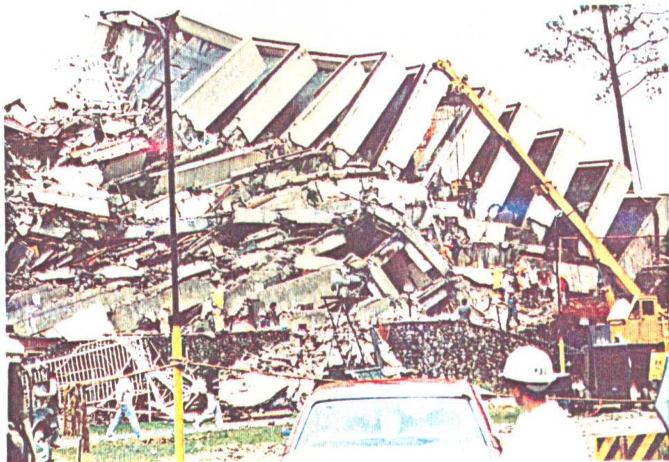
Photo 3.4 Brittle failure of the Hyatt Terraces hotel, 11-storey towers, typical misconceptual earthquake resistant design including other buildings in this hotel complex.
